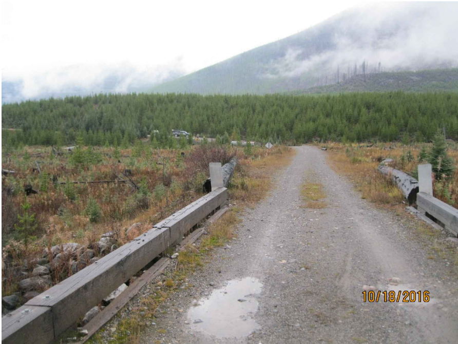
6 11 PHOTO 6 - EXISTING BRIDGE UP CHAINAGE SCALE: NTS
